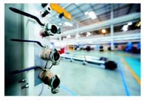
With seven manifold outlets installed at different points throughout the facility, compressed air is highly accessible when and where required.
